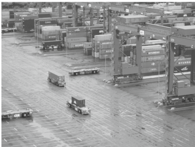
Fig. 10.6 Main driveways in front of ASC blocks at the HHLA Container Terminal Altenwerder
