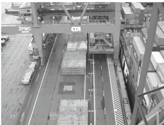
Fig. 10.3 Quay crane portal at the HHLA Container Terminal Altenwerder
