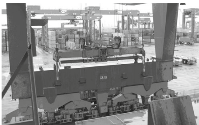
Fig. 10.1 Storage position for over height frame at the HHLA Container Terminal Altenwerder
