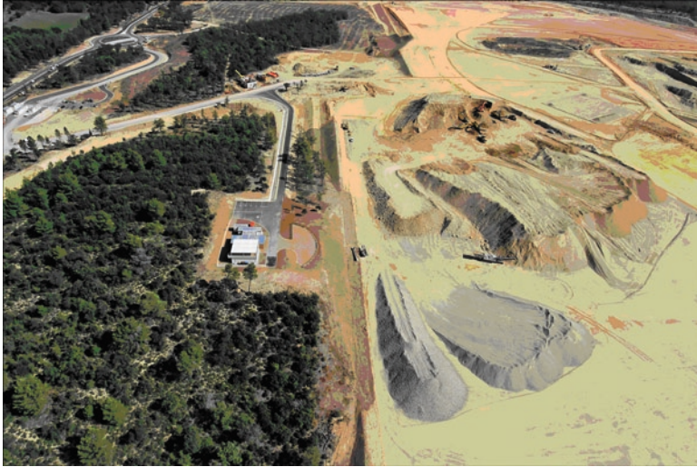
Fig. 8.26 Preparation of the ITER site in 2008
