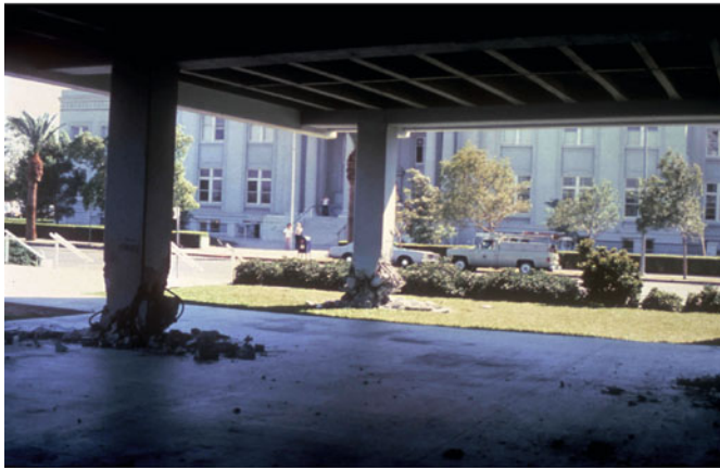
Earthquake Damage: Detection and Early Warning in Man-Made Structures, Figure 6 Imperial County Services (ICS) building: a view (towards north); b photographs of damage: columns F1 and F2 at the ground floor; and c column F1
