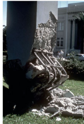
Earthquake Damage: Detection and Early Warning in Man-Made Structures, Figure 6 Imperial County Services (ICS) building: a view (towards north); b photographs of damage: columns F1 and F2 at the ground floor; and c column F1
