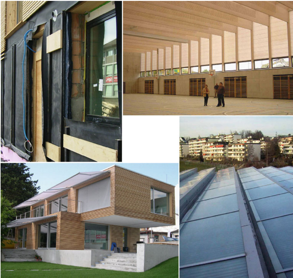
Figure 26.16. Examples of two aerogel insulation demonstration projects in Switzerland: Transparent insulation ( right , high-school gymnastic hall in Zürich) and façade blanket insulation ( left , single family home in Meilen, ZH).
