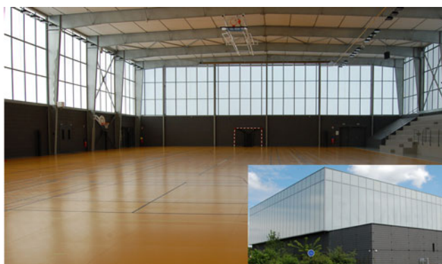
Figure 38.2. Cabot's aerogel in daylighting, Souchais Sports Complex, Carquefou, France.
