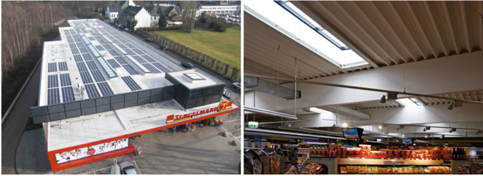
Figure 41.10. Left: The first low energy Supermarket “Tengelmann Klimamarkt” in Mühlheim an der Ruhr, Germany, with an 82 m 2 OKAGEL day-lighting system in the roof. Right: Vision from the inside showing the function of the daylighting system.
