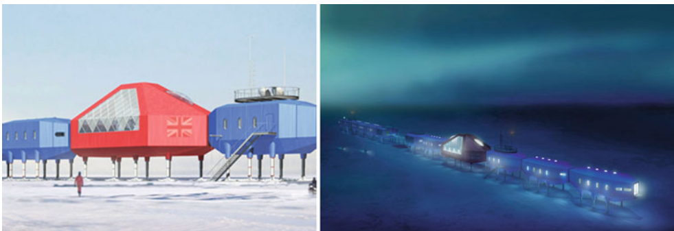
Figure 41.9. Left: Animation of the new British Antarctic Survey Research Station Halley VI. The red coloured main module contains 72 \text{ m}^2 OKAGEL as façade elements with an U -value of 0.3 \text{ W}/(\text{m}^2\text{K}) . Right: The entire research station at night.
