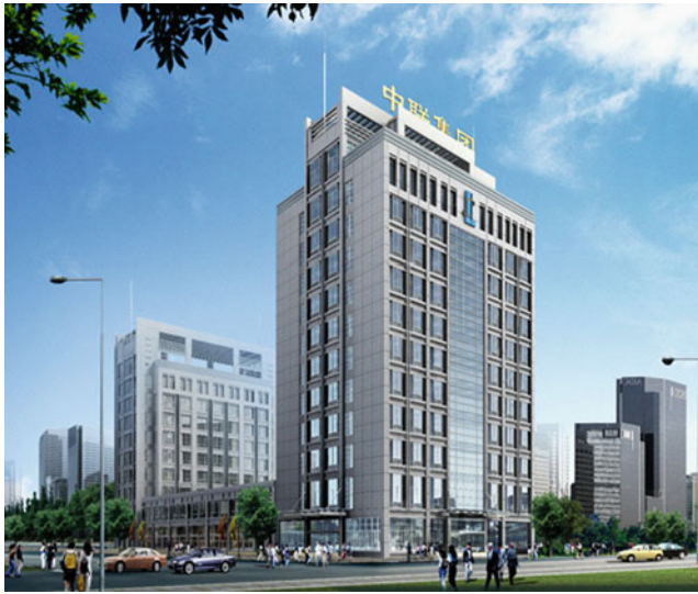
Figure 40.1. Office building of Nano High-tech.
