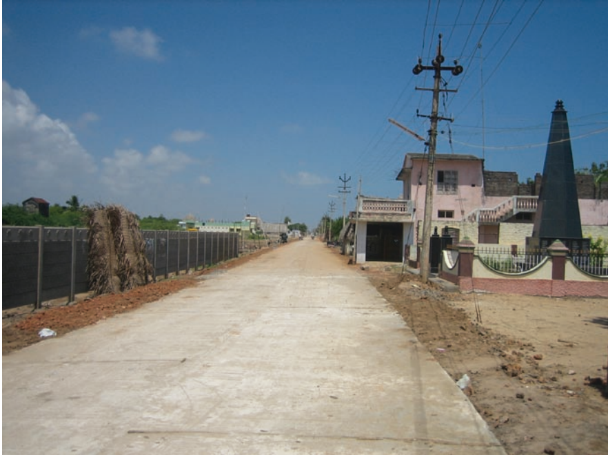
Fig. 6.1 The memorial monument to the right of a newly laid road. Photo by the author
