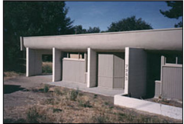
Passive Solar Heating in Built Environment. Figure 16 A mass roof: the Skytherm house in Atascadero California by Harold Hay (photo source: Evelyn and Harold Hay Fund at Cal Poly, San Luis Obispo, USA)
