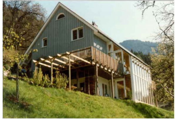
Passive Solar Heating in Built Environment. Figure 9 An Austrian passive solar house with solar air radiant heating and a sunspace in Nüziders, Vorarlberg (architect and photo source: Sture Larsen, www.solarsen.com )
