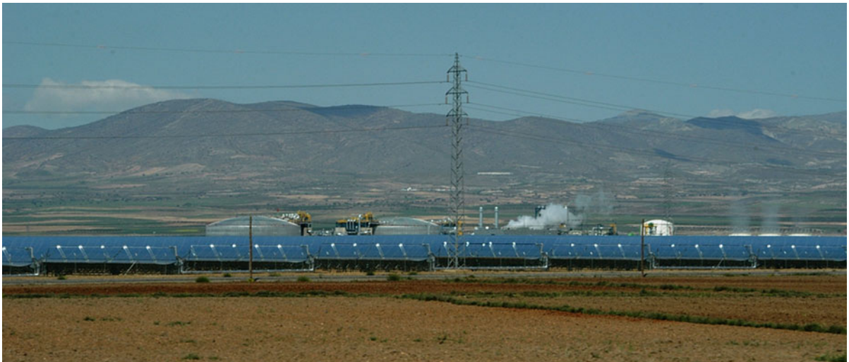
Parabolic Trough Solar Technology. Figure 6 Andasol-1 solar power plant in Granada (Spain)
