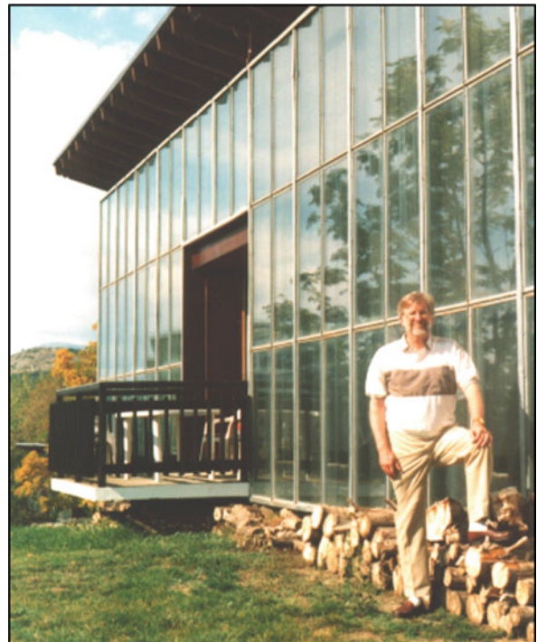
Passive Solar Heating in Built Environment. Figure 8 The Michel-Trombe wall house in Odello, FR (photo: robert.hastings@aeu.ch)
