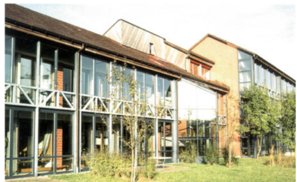
Passive Solar Heating in Built Environment. Figure 10 A Swiss school in Gumpenwiese ZH with sunspaces tied into the ventilation concept [16] (photo: robert.hastings@aeu.ch)
