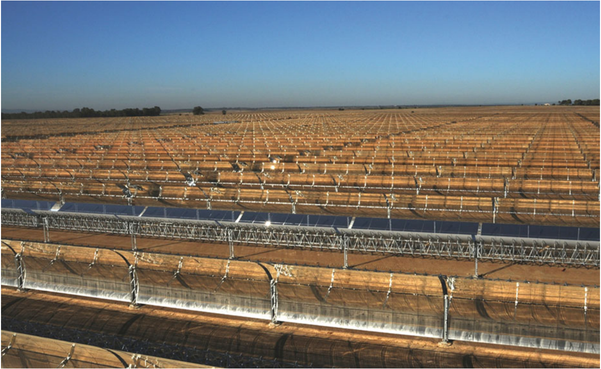
Parabolic Trough Solar Technology. Figure 7 Parabolic trough solar field, La Florida (Extremadura), Spain
