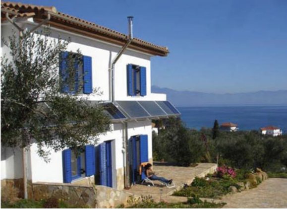
Passive Solar Heating in Built Environment. Figure 23 A solar air heater for a vacation home on a Greek island (photo and system information: www.grammer-solar-bau.de )
