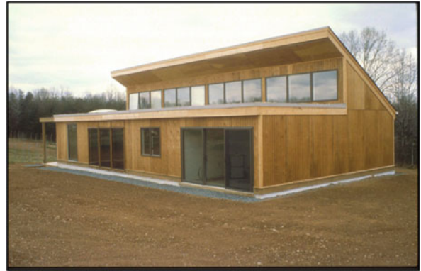
Passive Solar Heating in Built Environment. Figure 7 NBS (NIST) test house 1980, Gaithersburg, MD (architect and photo source: robert.hastings@aeu.ch)
