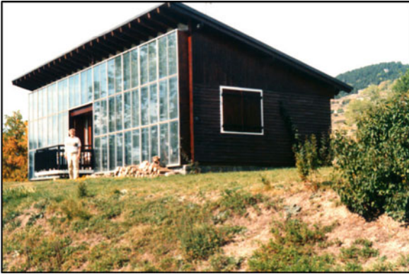
Passive Solar Heating in Built Environment. Figure 15 The prototype Michel-Trombe wall house in Odeillo, FR (source: Robert.hastings@aeu.ch)
