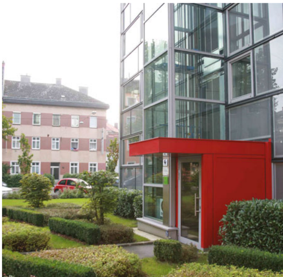
Passive Solar Heating in Built Environment. Figure 20 Apartment building with the GAP solar insulation on Makartstraße, Linz AT (photo source: S. Grünewald and S. Rottensteiner)
