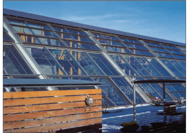
Passive Solar Heating in Built Environment. Figure 26 Attached sunspaces as part of the concept of low energy row housing in Bern (Architects, AARPLAN; Bern, CH)
