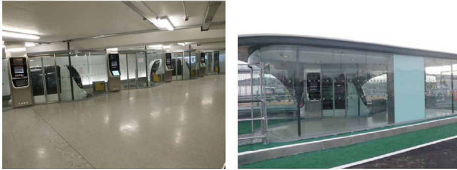
Personal Rapid Transit and Its Development. Figure 11 Two Heathrow Station Design (Martin Lowsen of ULTra)
