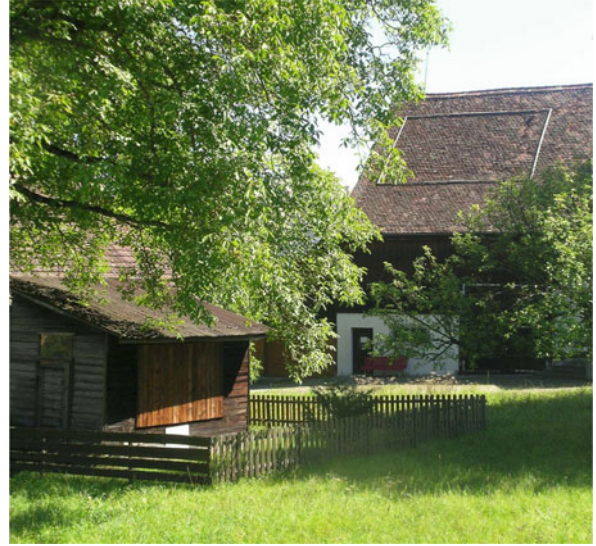
Passive Solar Heating in Built Environment. Figure 11 Renovation with solar and conservation, 60 examples of projects across Europe and Canada [17]
