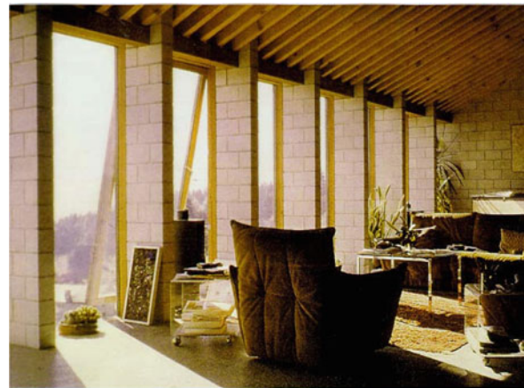
Passive Solar Heating in Built Environment. Figure 13 Extreme example of a direct-gain house in Trin/CH with no auxiliary heating (architect Andrea Ruedi, CH-7000 Chur)
