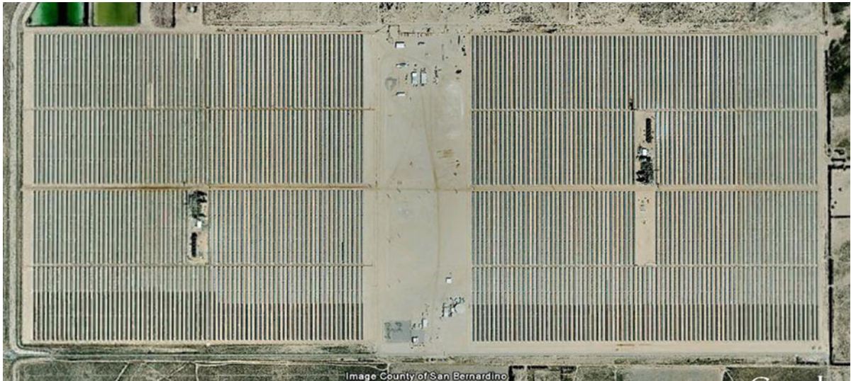
Parabolic Trough Solar Technology. Figure 13
