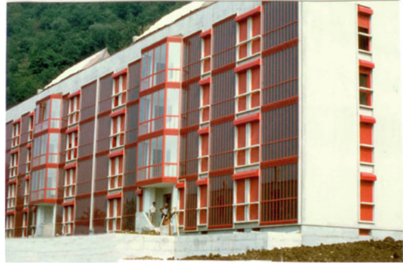
Passive Solar Heating in Built Environment. Figure 25 Solar apartment buildings in Marostica by Barra Costantini (photo: Gianni Scudo)
