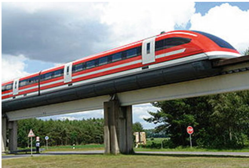
MAGLEV Technology Development. Figure 38 Transrapid 09 at the Emsland test facility in Germany
