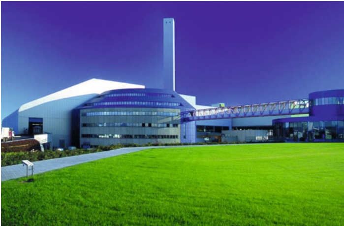
Martin Waste-to-Energy Technology. Figure 43 Brescia (IT)
