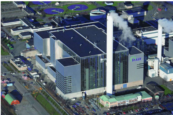
Martin Waste-to-Energy Technology. Figure 44 Malmö (SE)
