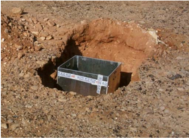
Fig. 17.1 Protection steel box (uncovered) in a dug hole.
