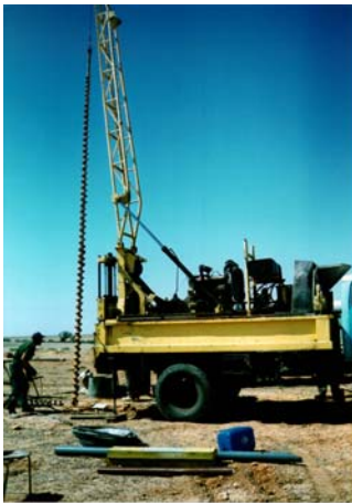
12 m deep test borehole
