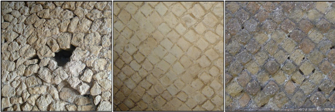
Architecture, Roman, Fig. 3 Examples of opus incertum in the Sanctuary of Jupiter Anxur in Terracina, of early opus reticulatum in the Theater of Pompey in
