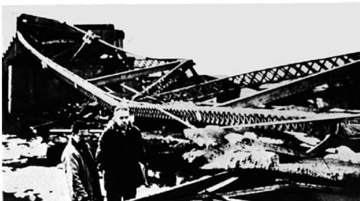
Fig. 1.3 On December 15, 1967, the Silver Bridge connecting Ohio and West Virginia over the Ohio River collapsed, and 46 people lost their lives. The cause of the collapse was stress-corrosion cracking [3]
