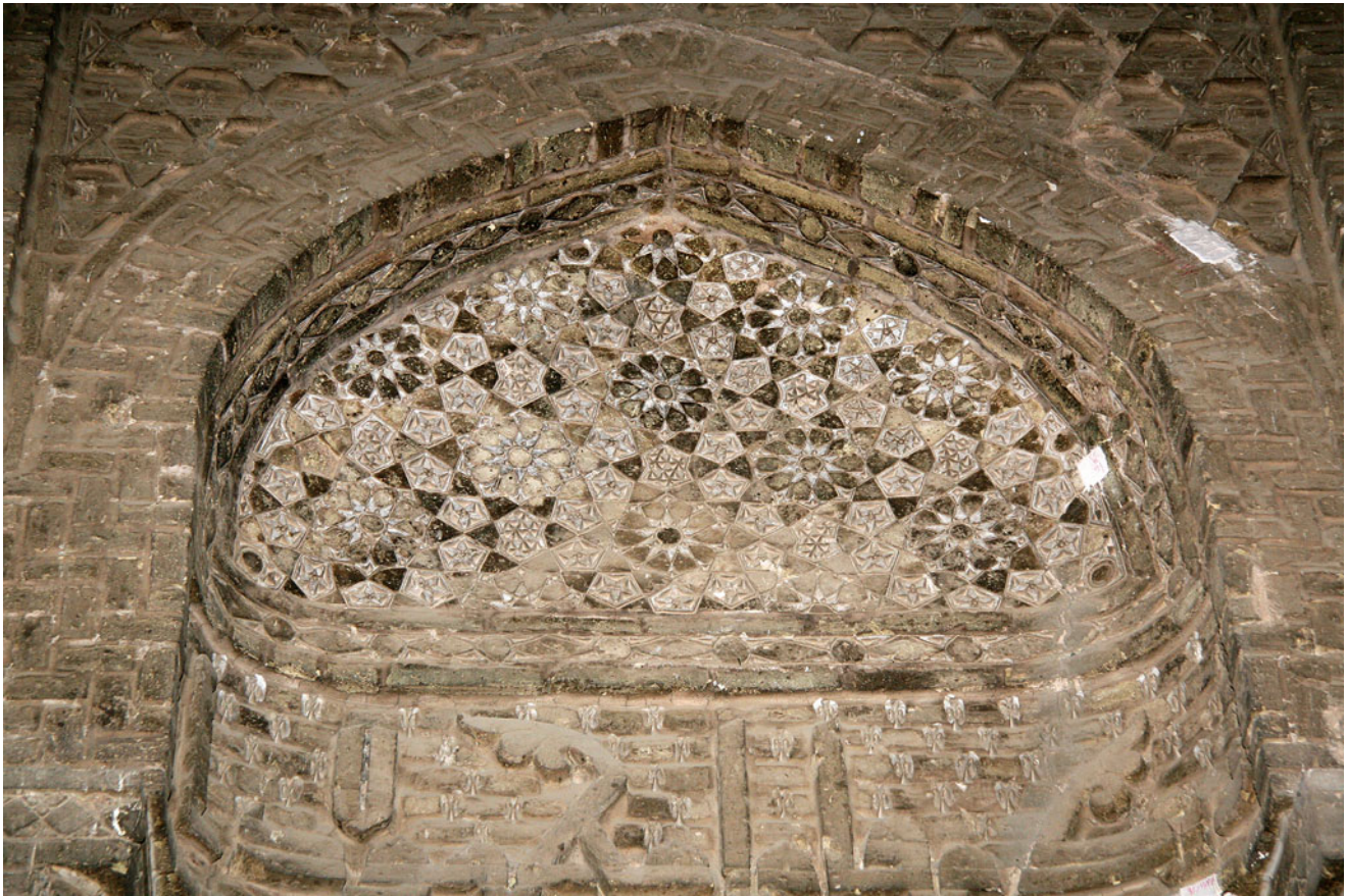
Photograph 21 A Seljuk example of the classic obtuse pattern with ten-pointed stars created from the fivefold system in the northeast dome chamber of the Friday Mosque at Isfahan (© Tom Goris)
