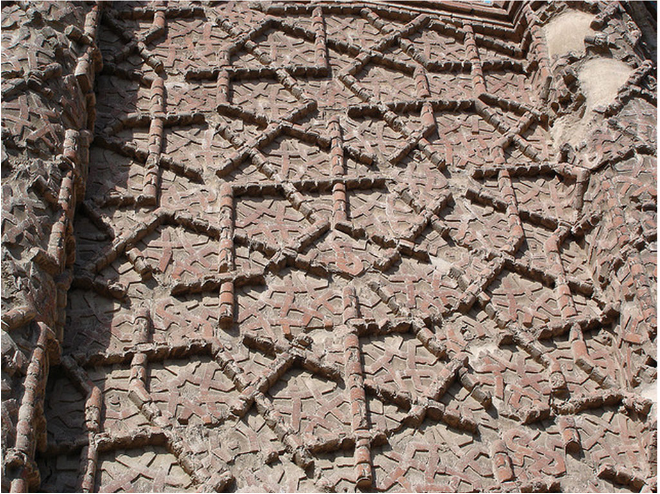
Photograph 24 A Seljuk dual-level design from the façade of the Gunbad-i Qabud in Maragha, Iran, wherein the primary pattern is created from the fivefold system (© Richard Mortel)
