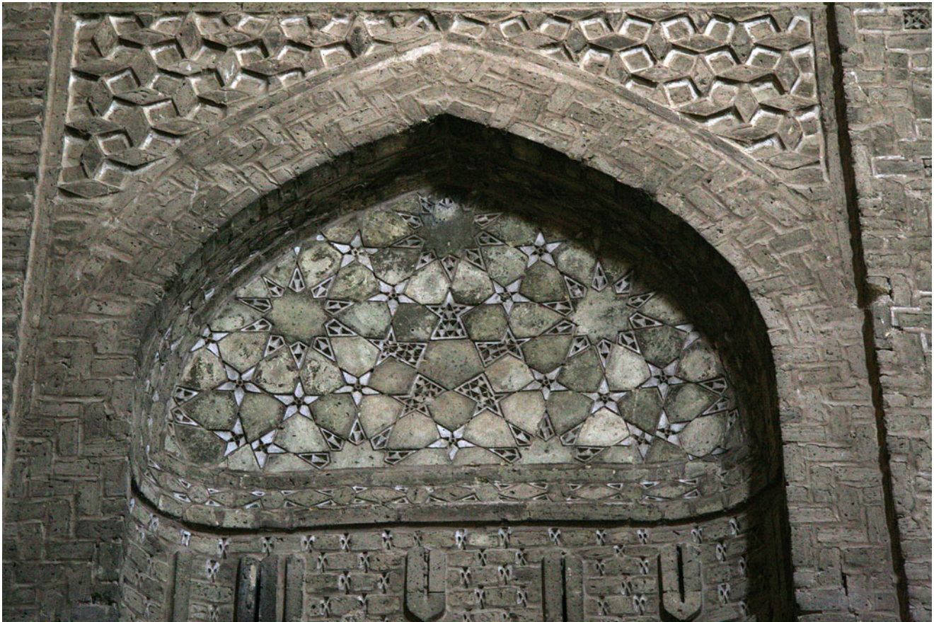
Photograph 25 A Seljuk hybrid acute design with ten-pointed stars created from the fivefold system in the northeast dome chamber of the Friday Mosque at Isfahan (© Tom Goris)
