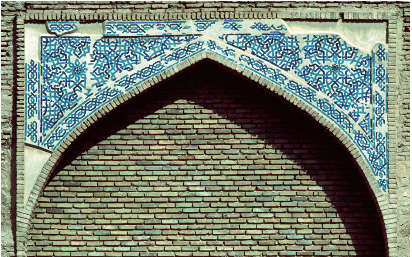
Photograph 68 An Ilkhanid cut-tile mosaic and stucco arch spandrel from the mausoleum of Uljaytu at Sultaniya, Iran, with a nonsystematic additive two-point pattern (© David Wade)
