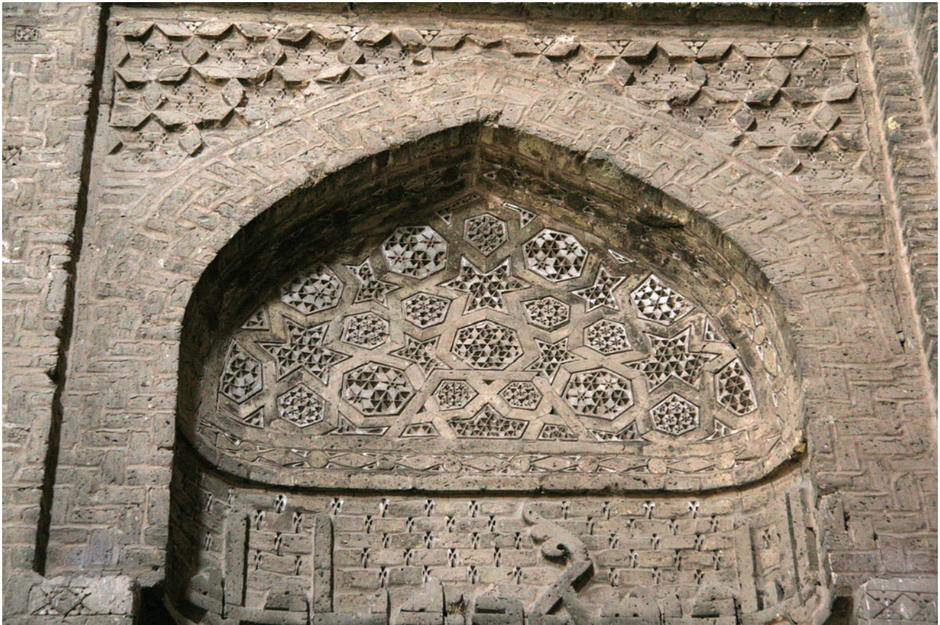
Photograph 27 A Seljuk nonsystematic threefold acute pattern with six-pointed stars and heptagons in the northeast dome chamber of the Friday Mosque at Isfahan (© Tom Goris)
