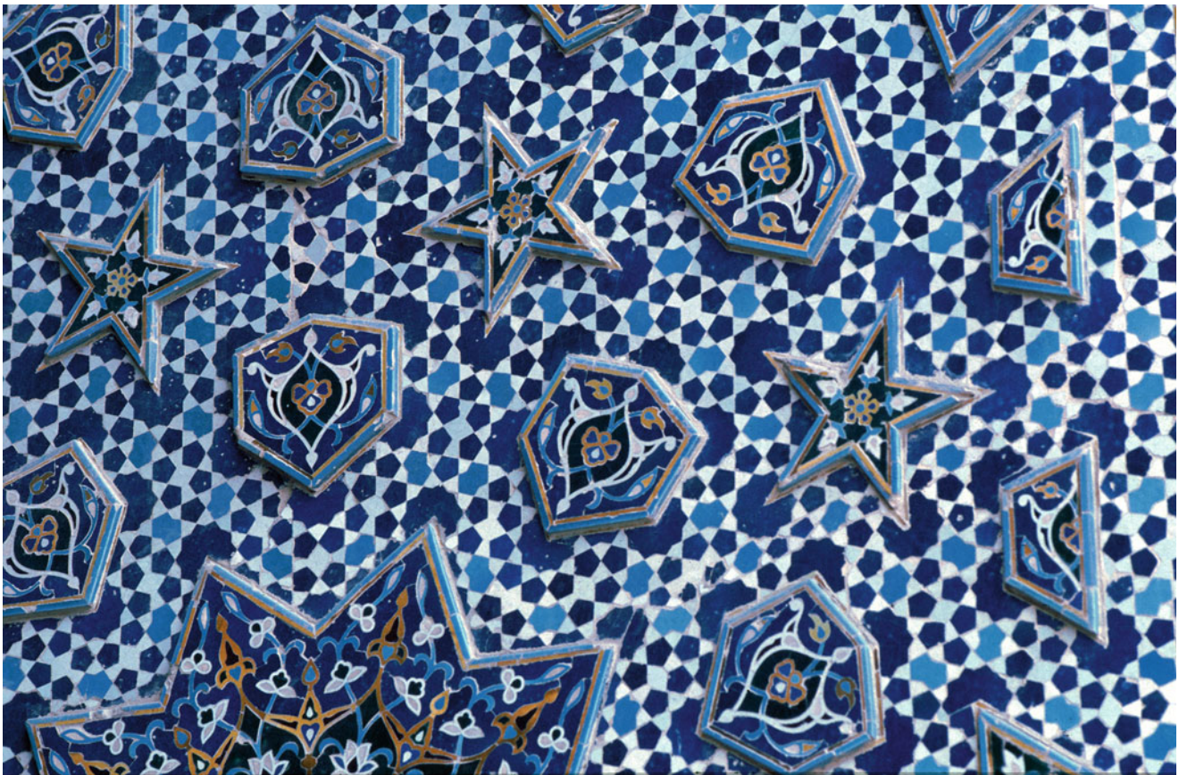
Photograph 98 A Qara Qoyunlu cut-tile mosaic panel at the Imamzada Darb-i Imam in Isfahan that employs a type B self-similar dual-level design that is constructed from the fivefold system (© David Wade)
