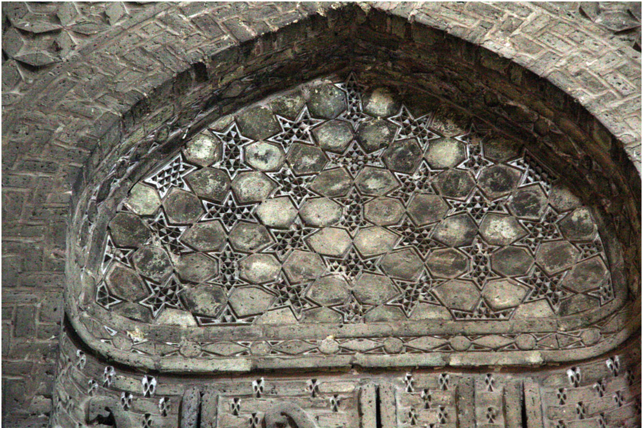
Photograph 26 A Seljuk acute pattern created with underlying modules included in the sevenfold system from the northeast dome chamber of the Friday Mosque at Isfahan (© Tom Goris)
