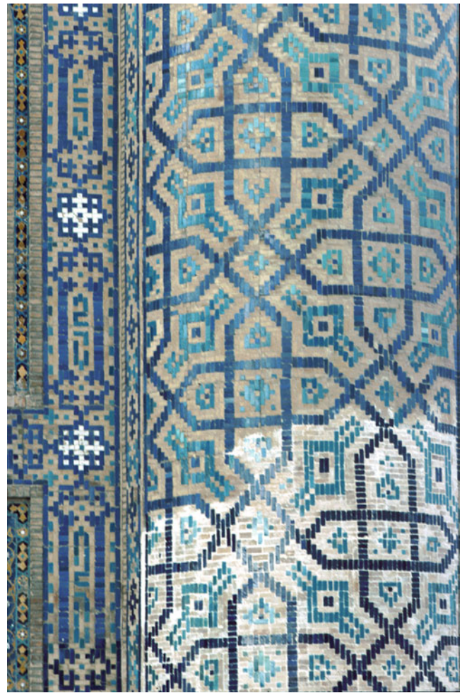
Photograph 71 Shaybanid polychrome brickwork from the Tilla Kari madrasa in Samarkand with a median pattern created from the fourfold system A (© David Wade)
