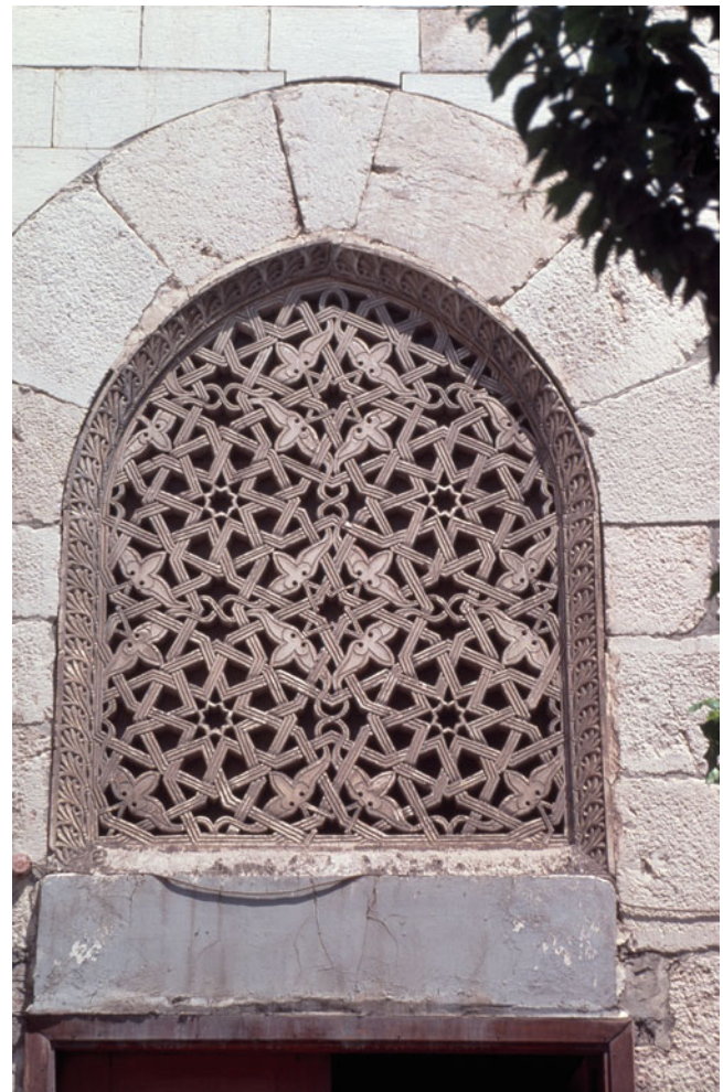
Photograph 37 A Zangid window grille at the Nur al-Din Bimaristan in Damascus with a fourfold median pattern created with the fourfold system A (Photo by Nasser Rabbat, courtesy of the Aga Khan Documentation Center at MIT)
