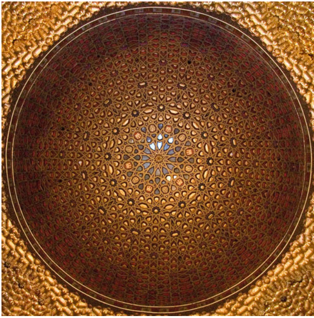
Photograph 67 The Mudéjar dome over the Hall of Ambassadors in the Alcázar of Seville with an acute pattern produced from the fivefold system (© Jean-Guillaume Dumont)
