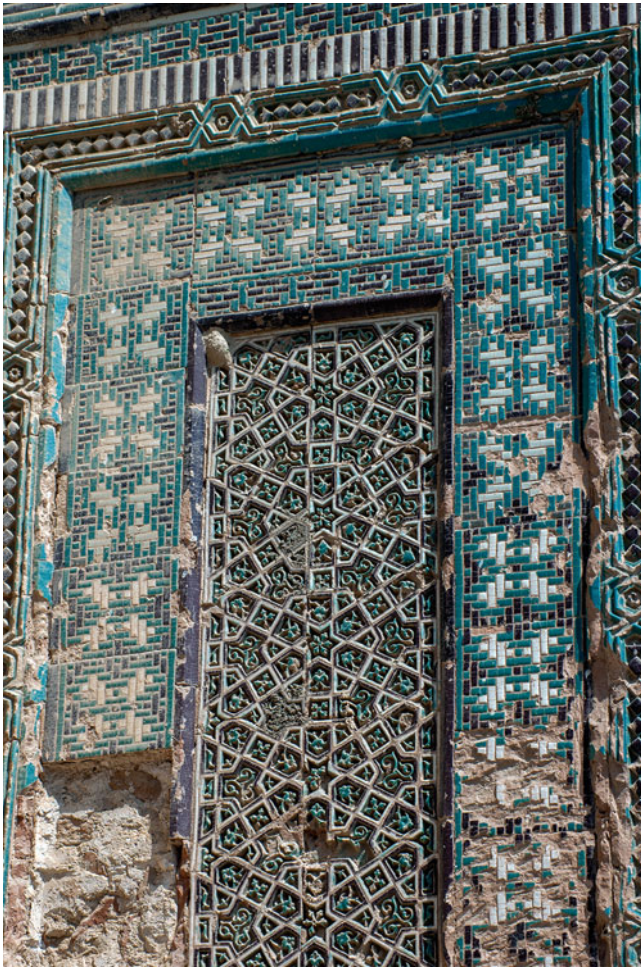
Photograph 70 A Chaghatayid ceramic panel from the mausoleum of Tughluq Temür in Huocheng, western China, with a two-point pattern that is easily constructed with the system of regular polygons (© Daniel C. Waugh)
