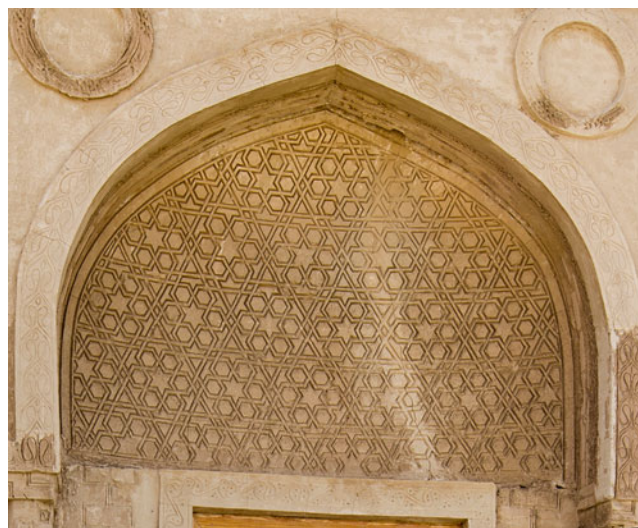
Photograph 12 A Samanid threefold pattern with six-pointed stars easily created from the system of regular polygons in the tympanum over the pishtaq of the mausoleum of Arab Ata in Tim, Uzbekistan (© Bernard O’Kane)
