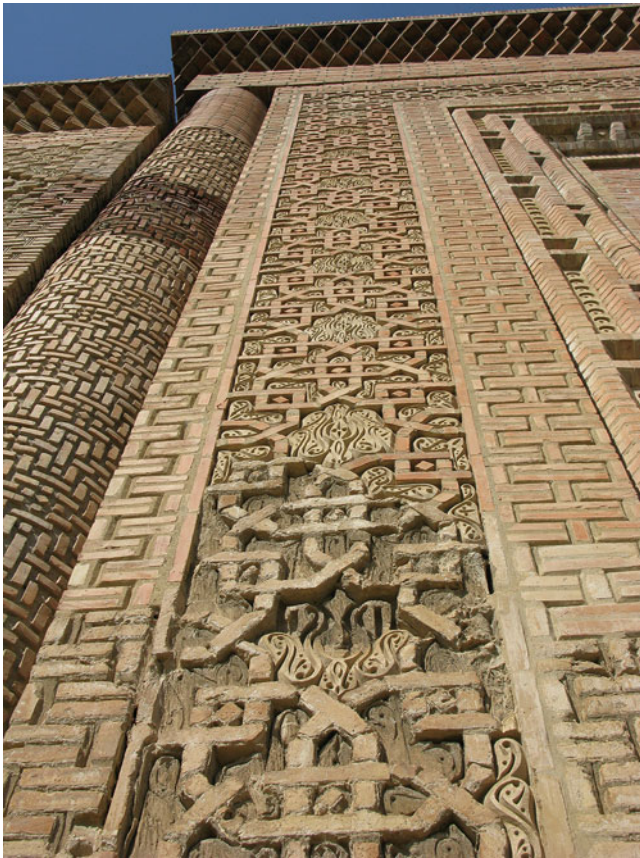
Photograph 15 A Qarakhanid raised brick pattern with eight-pointed stars created from the fourfold system A in the entry façade of the tomb of Nasr ibn Ali in Uzgen, Kyrgystan (© Igor Goncharov)
