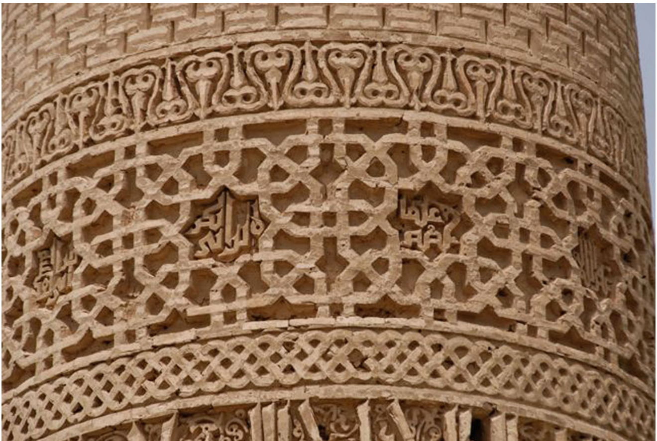
Photograph 20 A Seljuk example of a pattern with eight-pointed stars created from the fourfold system A on the minaret of Daulatabad outside Balkh, Afghanistan (© Thalia Kennedy)
