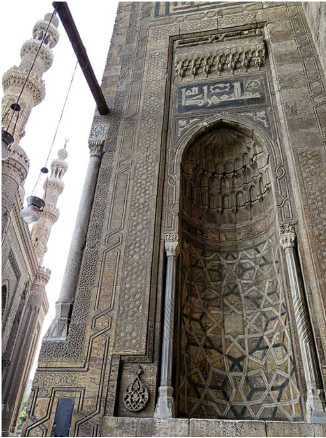
Photograph 58 A Mamluk niche in the entry portal of the Sultan al-Nasir Hasan funerary complex in Cairo with a nonsystematic pattern that includes its underlying generative tessellation, as well as a nonsystematic border pattern that surrounds the niche (© Scott Haddow)
