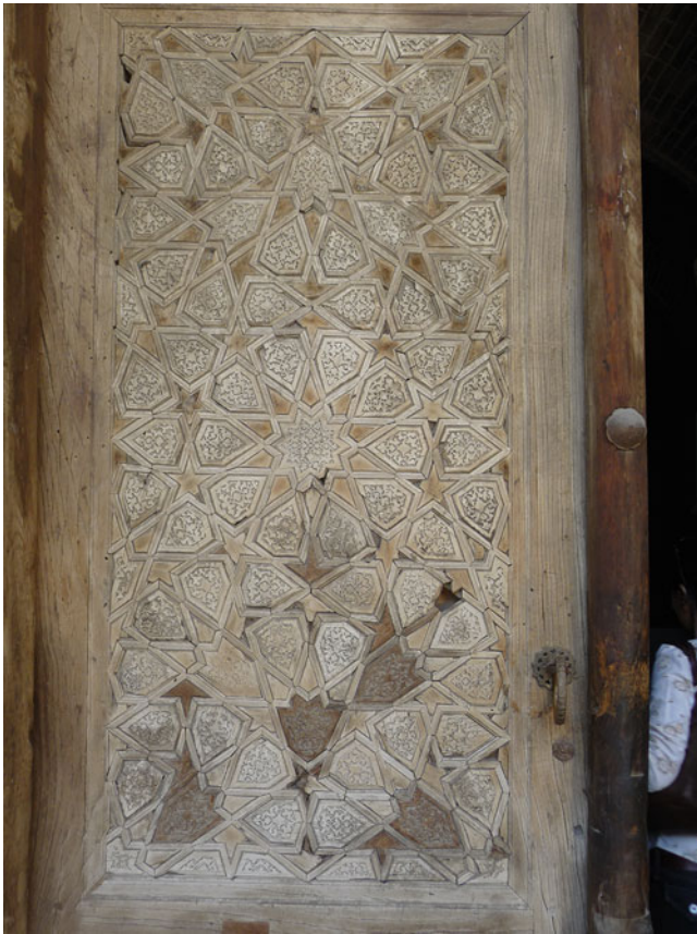
Photograph 78 Shaybanid wood joinery from a door panel at the Kukeldash madrasa in Bukhara, Uzbekistan, that employs an acute pattern created from the fivefold system (© Thalia Kennedy)
