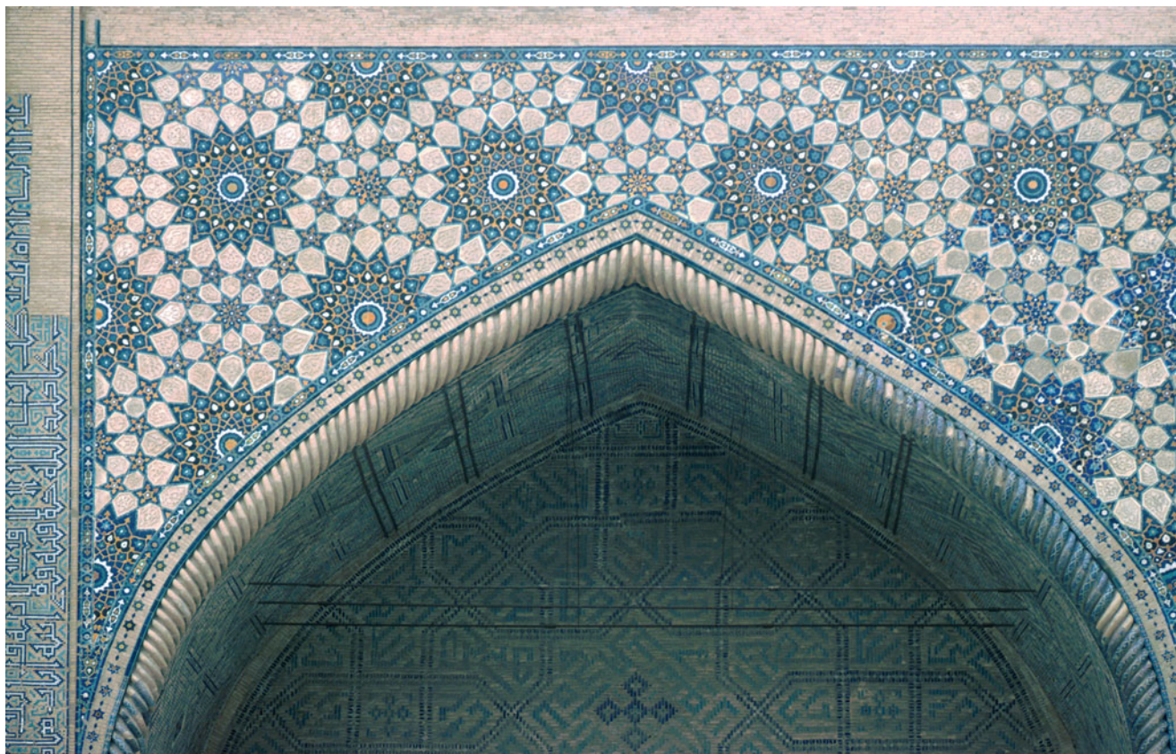
Photograph 89 A Timurid cut-tile mosaic arch spandrel at the Ulugh Beg madrasa in Samarkand that employs a nonsystematic acute pattern made up of 8- and 16-pointed stars (© David Wade)
