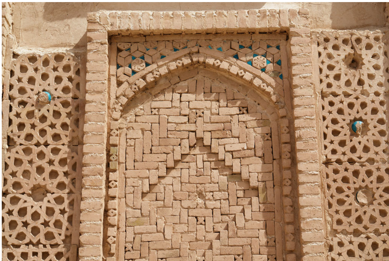
Photograph 23 Seljuk unglazed brick and terra-cotta geometric ornament from the exterior façade of the Friday Mosque at Gonabad, Iran (photograph by Farshid Emami; courtesy of the Aga Khan Documentation Center at MIT)
