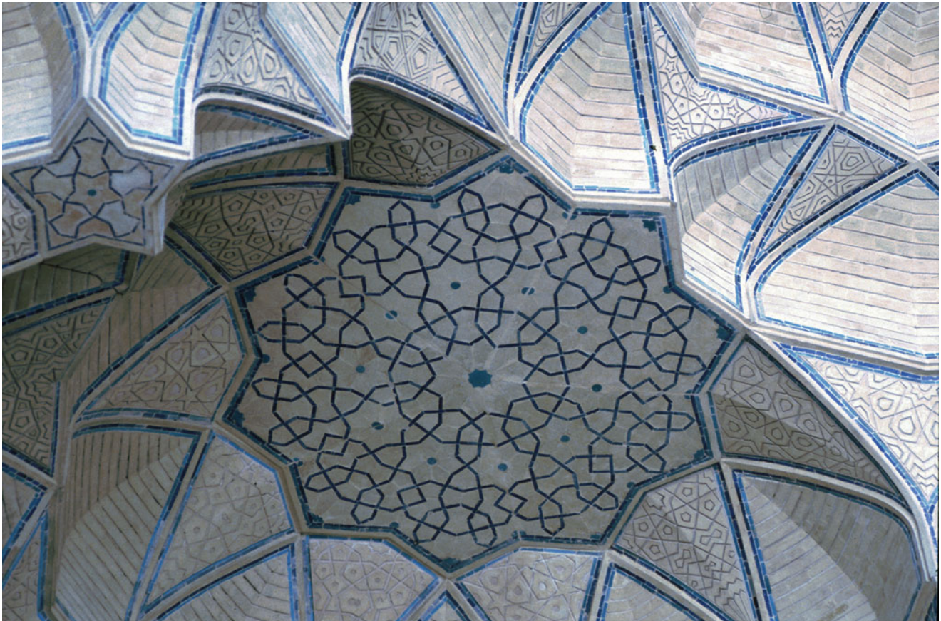
Photograph 90 Detail of a ten-pointed star soffit from the Safavid muqarnas in the southeast iwan of the Friday Mosque at Isfahan that employs a nonsystematic radial median pattern with seven- and ten-pointed stars (© David Wade)
