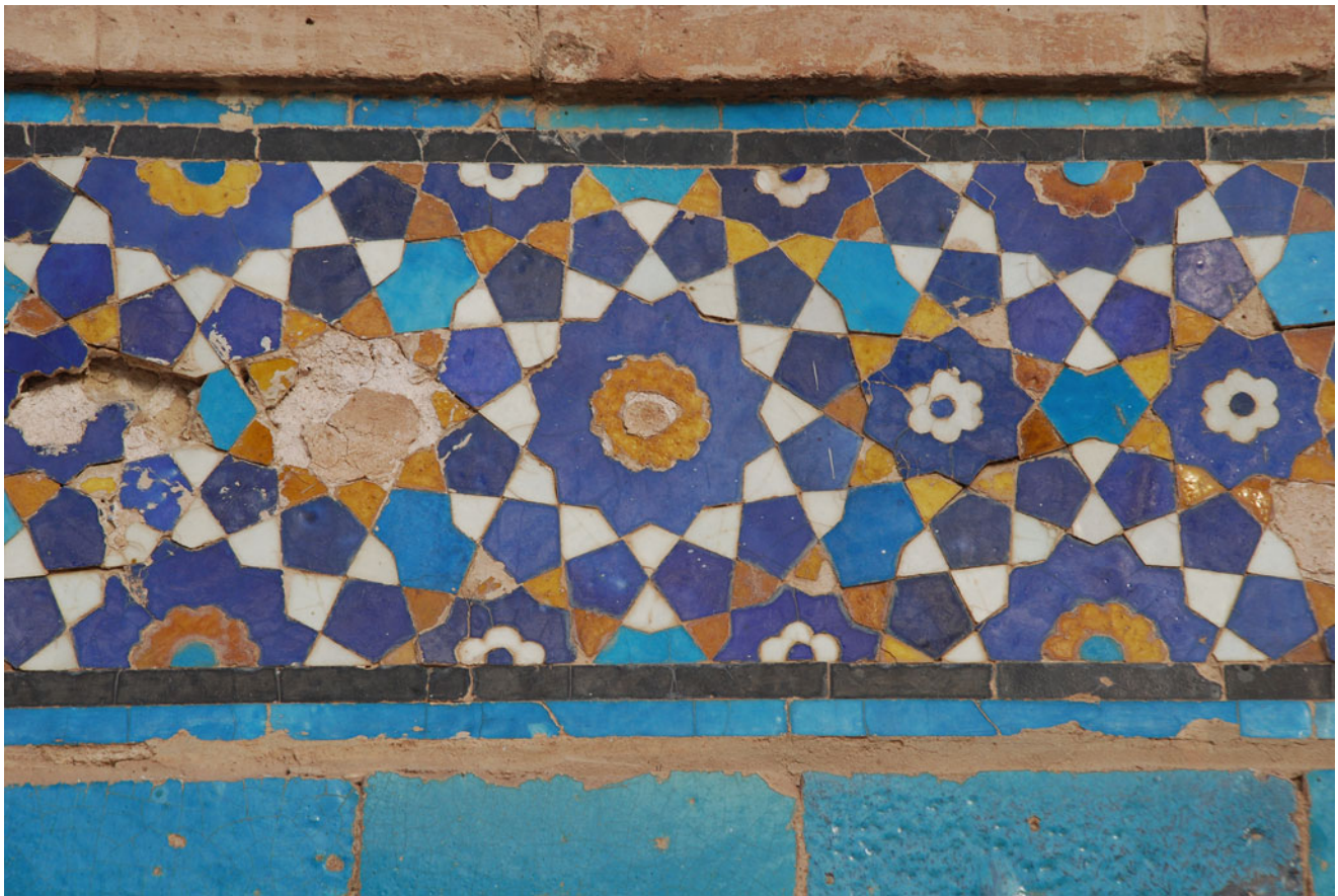
Photograph 85 A Timurid cut-tile mosaic border at the Abdulla Ansari complex in Gazargah, Afghanistan, that employs a nonsystematic threefold obtuse pattern with 9- and 12-pointed stars (© Thalia Kennedy)
