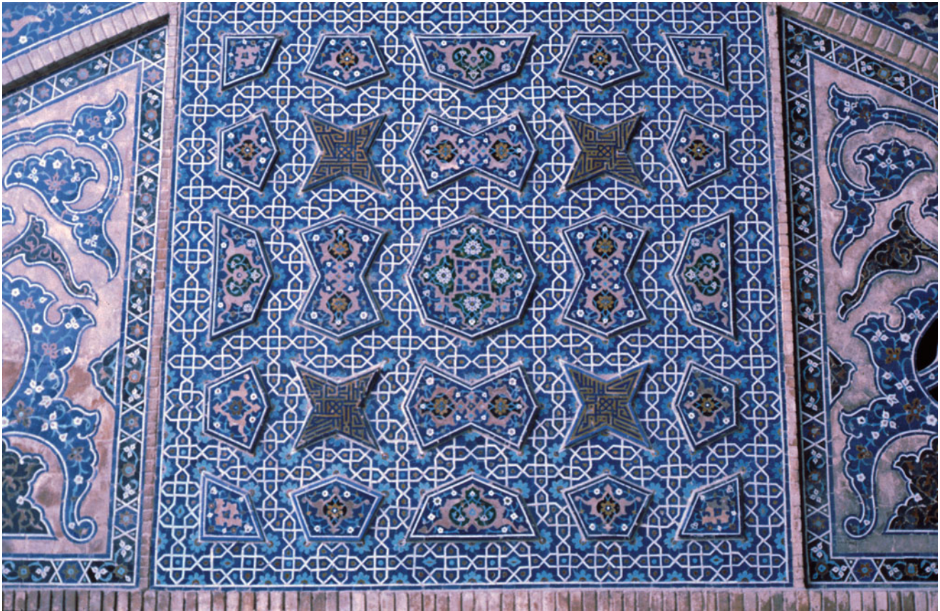
Photograph 99 An Aq Qoyunlu cut-tile mosaic panel from the Friday Mosque at Isfahan that employs a type B dual-level design that is constructed from the fourfold system A (© David Wade)
