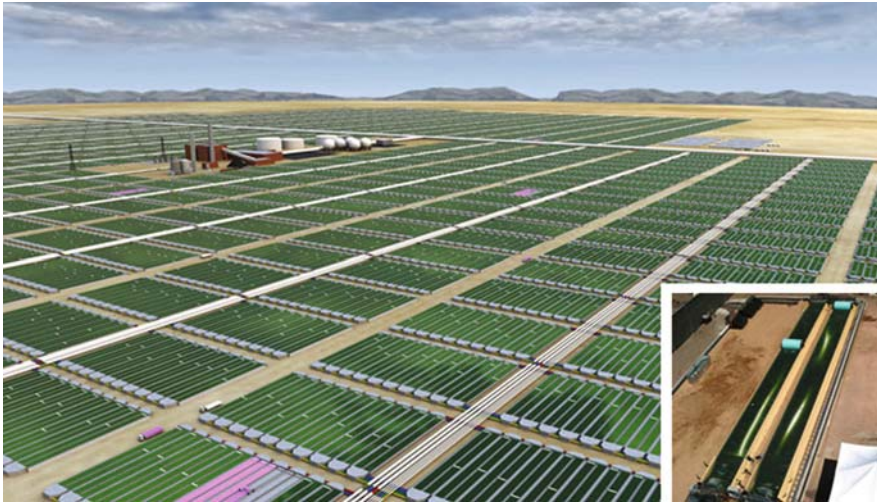
Fig. 9.6 Colorado's Solix Biofuels tackles the difficult task of harvesting algae for oil with a field of bioreactors that take a kind of painter's drop cloth (inset) to bubble CO through its system. From Popular Mechanics online article "Pond-Powered Biofuels: Turning Algae into America's New Energy" 2007 ( http://www.popularmechanics.com/science/earth/4213775.html )
