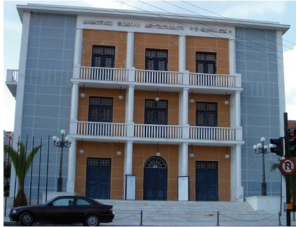
Fig. 6.18 Façade of theatre building with the two walls chosen for strengthening in shear with FRP
