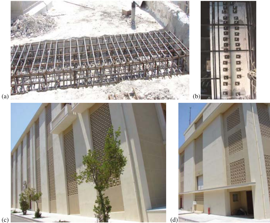
Fig. 6.15 Features of the retrofitting of the theatre building: (a) RC belt straddling joint at roof level; (b) steel rods connecting interior walls across the joint; (c) long side of the building with finished wall jackets; (d) new bay-long walls at the back
