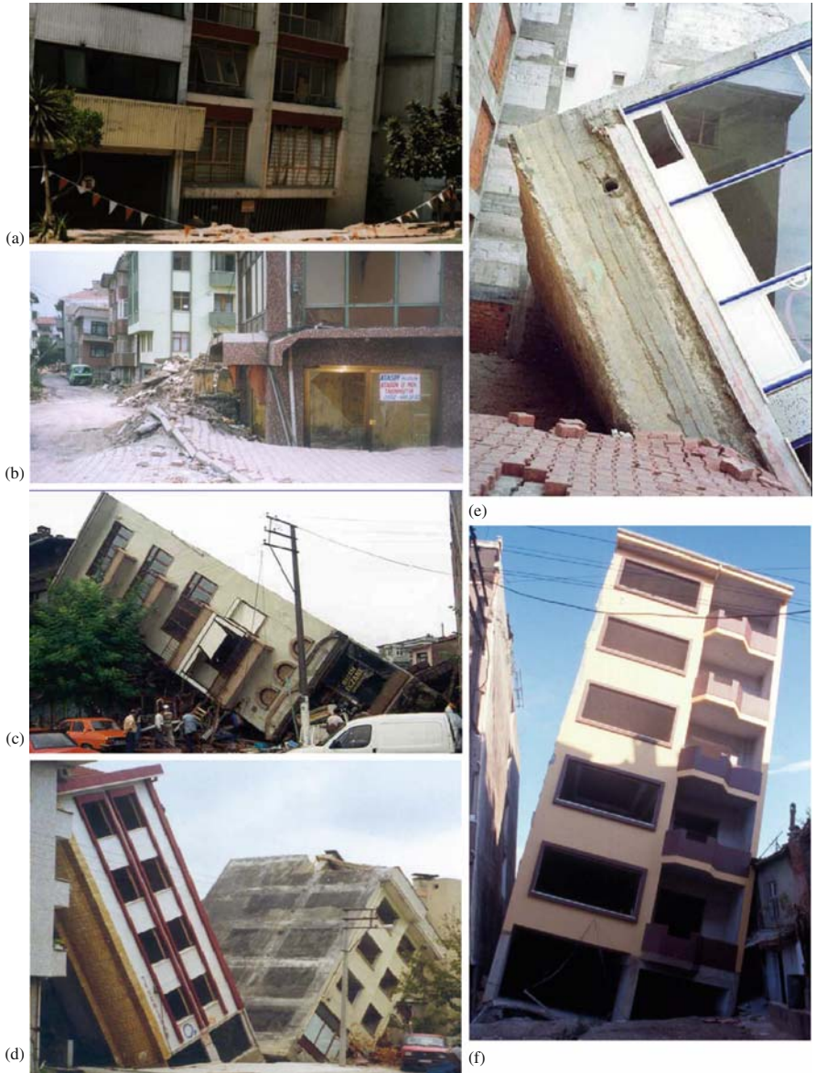
Fig. 2.18 Bearing capacity failures at: (a) in Mexico City (1985) (b)–(f) Adapazari (TR) in the 1999 Kocaeli earthquake (courtesy G. Gazetas, NTUA). (See also Colour Plate 6 on page 720)
