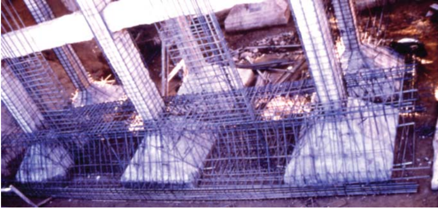
Fig. 6.7 New wall founded on foundation beam encapsulating footings of nearby columns
