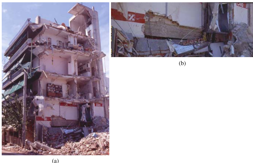
Fig. 2.23 Apartment building in Athens: (a) wing that did not collapse; (b) detail of (a) showing the side of the 1st storey beam along the line where floor diaphragms were torn apart
