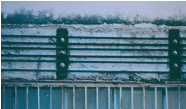
Plate 16 Collector element of the wall in Fig. 6.5, fastened to the side of the perimeter beam (See also Figure 6.6 on page 670)
