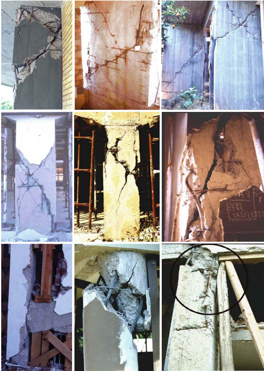
Fig. 3.35 Shear failures of columns or walls (See also Colour Plate 9 on page 723)
