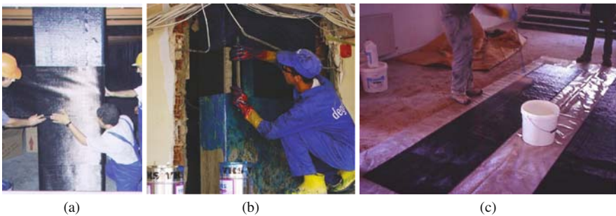
Fig. 6.3 Hand lay-up of FRPs in situ: (a), (b) dry fabric impregnated in place (courtesy A. Ilki); (c) impregnation of the fabric right before placing (See also Colour Plate 15 on page 729)
