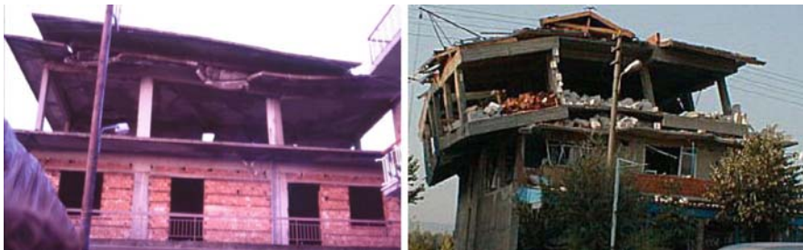
Fig. 2.3 Collapse of upper storeys with reduced plan dimensions ( left ): Kalamata (GR) 1986; ( right ): Kocaeli (TR) 1999
