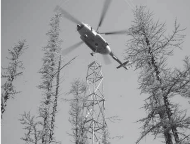
Fig. 10.1 A helicopter transporting the wooden tower to the study site. The tower was landing on the ground (Photo: Y. Matsuura)
