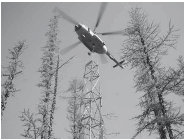
Fig. 10.1 A helicopter transporting the wooden tower to the study site. The tower was landing on the ground (Photo: Y. Matsuura)
