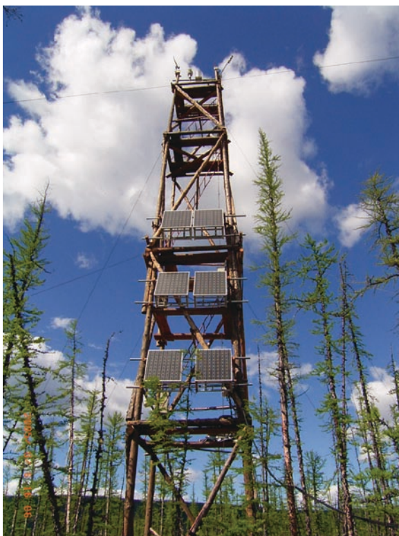
Fig. 10.2 The tower equipped with all devices (Photo: Y. Nakai)
