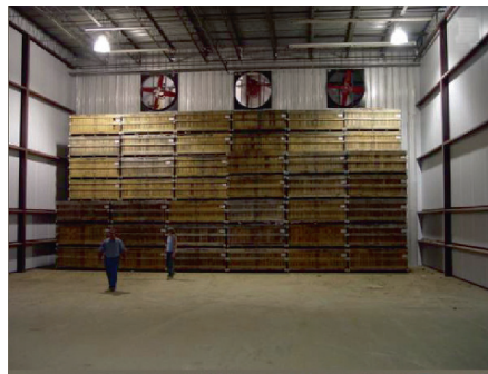
Plate 11 Commercial grower-shipper bulk bin storage room equipped with environmental management controls, Nash County, North Carolina (See also Plate 13.2 on page 275)
