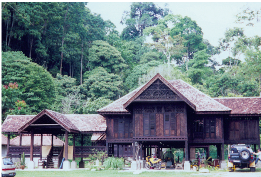
Fig. 1.1 Janda Baik zawiya (Sufi lodge)
