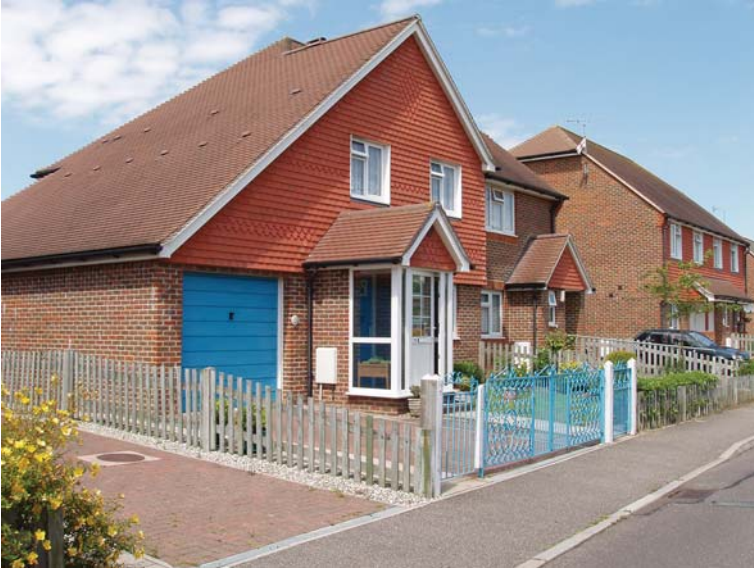
Fig. 9.7 Cooper Road, East Sussex
