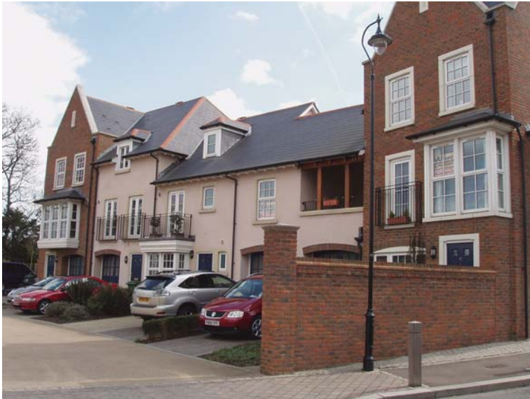
Fig. 9.9 Ingress Park, Kent
