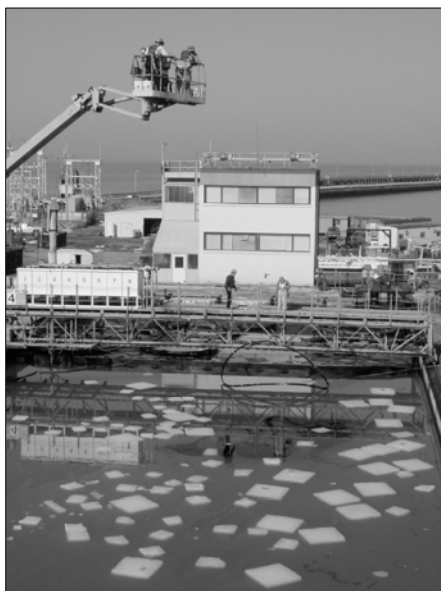
Figure 16. Containment ring lifted to release oil to drift into ice.
