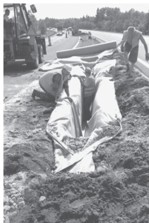
Fig. 13.15 Trench drain (a) without pipe, (b) with pipe, (c) in central reserve 2 . (Credit: B. Gajewska)
