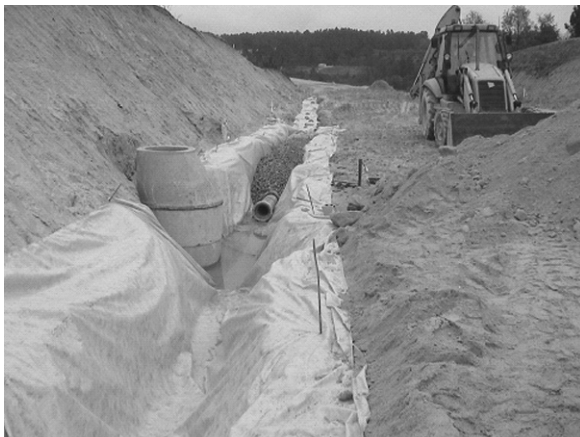
Fig. 13.14 Constructing of a trench (French) drain
