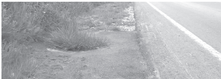
Fig. 13.44 Sometimes drainage problems can be seen easily and from the surface
