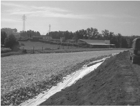
Fig. 13.19 Drainage layers
