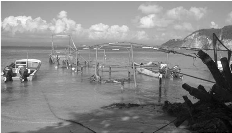
Fig. 10 Destroyed berth in Petit Havre
