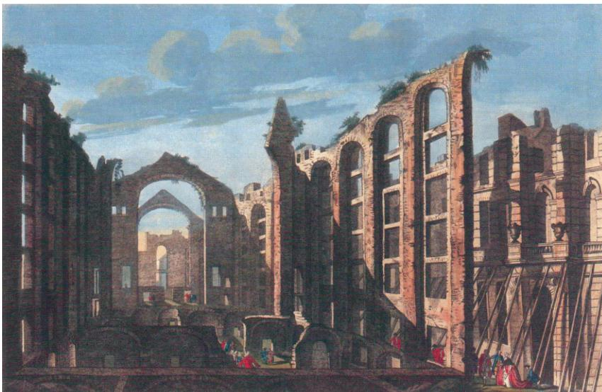
Fig. 16 Structure with slender walls without falling (Opera House or Real Theater) denoting damage caused essentially by the fire
