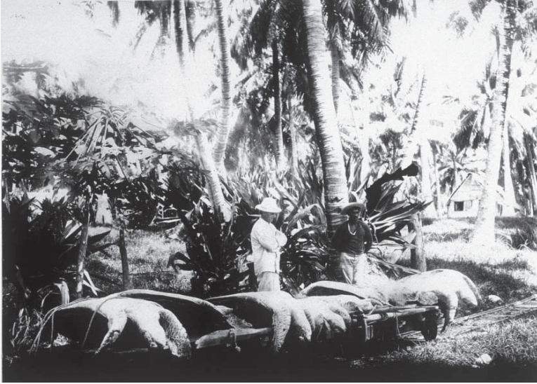
FIG. 15.19. Hand-hauled rail trucks carry guano, copra, timber and large green turtles in this anonymous 1908 photo taken at Flint Is. (Photo courtesy of the Mary Lea Shane Archives, Lick Observatory, University of California, Santa Cruz)
