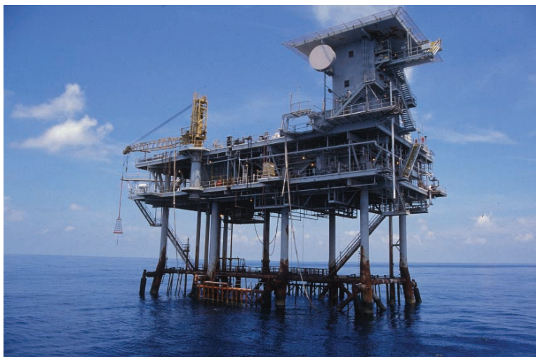
FIG. 6.28. A natural gas production platform, High Island A389A, located within the boundaries of the East Flower Garden Bank, less than 2 km from the coral reef crest (Photo credit: FGBNMS/G.P. Schmahl)
