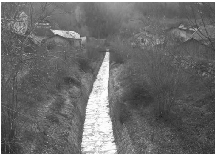
Figure 12: Trapezoidal Channel through the Village (construction: 1974–1975).
