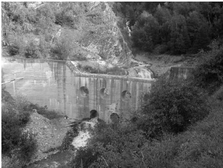
Figure 11: Debris Retention Basin Immediately Upstream of the Village (construction: 1973)
