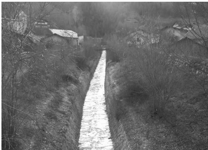
Figure 12: Trapezoidal Channel through the Village (construction: 1974–1975).
