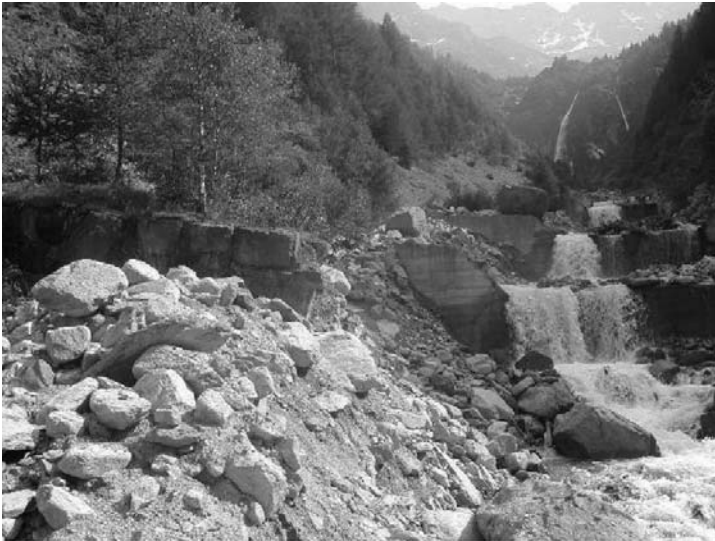
Figure 10: Check Dam Series in the Transition Zone of the Torrent (construction: 1972–1973).
