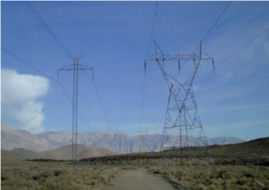
Figure 3. Comparison Left, power line: HVDC, 3,000 MW, \pm 500 kV bipole. Right, high voltage AC 400 MW line. (Pacific Direct Current Intertie PDCI near Bishop, CA)
