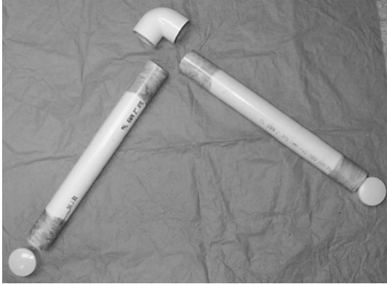
Step 1. Primed pieces of PVC pipe and fittings ready to be glued
