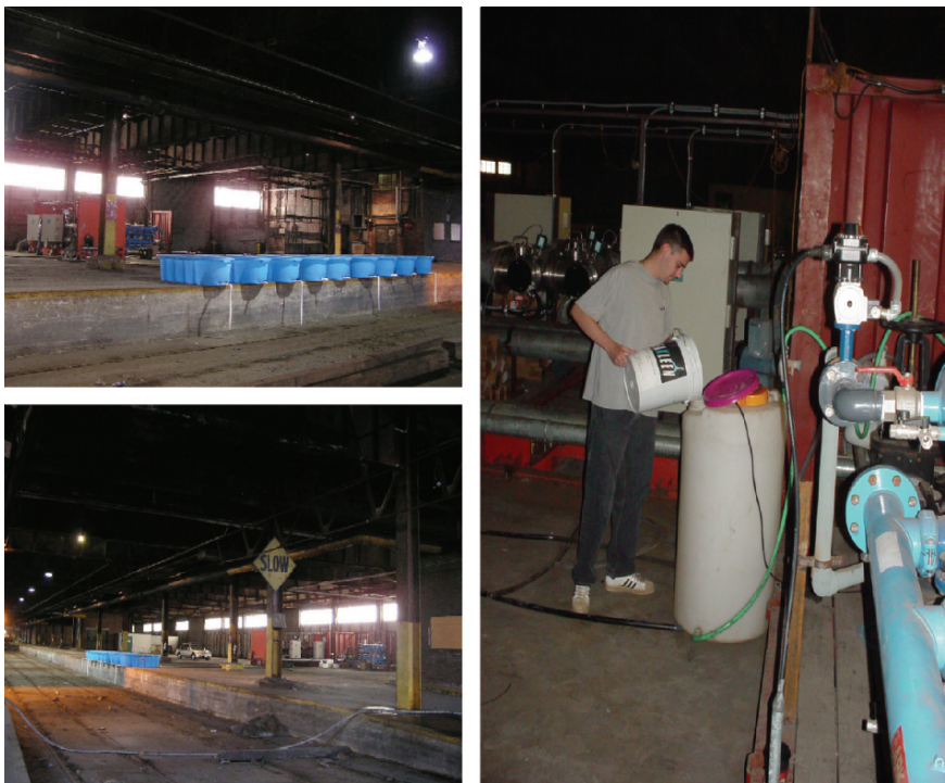
Fig. 1 Baltimore Ballast Water Treatment Technology Testing Facility (Maryland Port Administration, Clinton St. Terminal). Tank layout and biocide dosing equipment.
