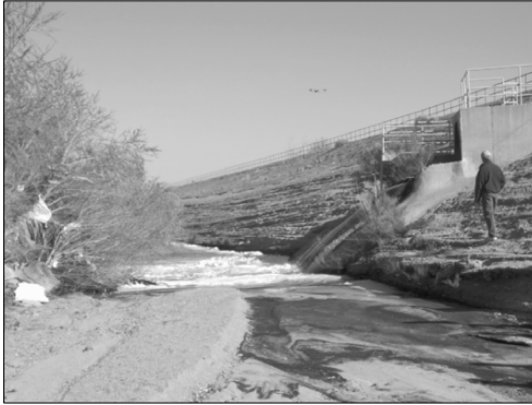
Figure 2. Outfall of regional wastewater treatment facility (Courtesy of Pima County Regional Flood Control District.)
