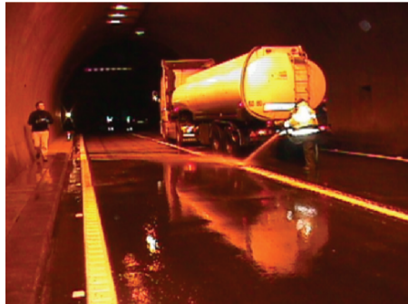
Fig. 2. View of the tunnel 2nd wash operation
