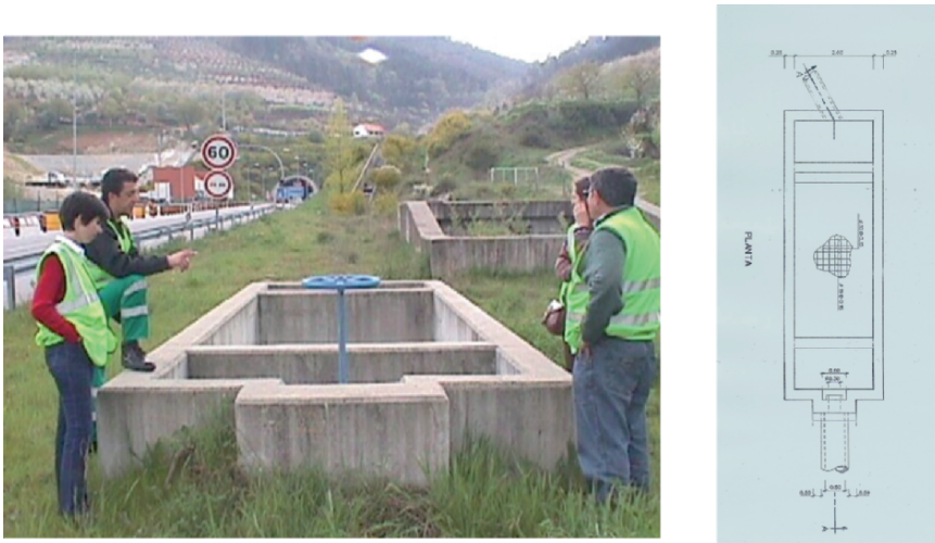
Fig. 1. View of the tunnel and of the collecting oil separator tank
