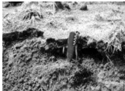
Photo 6. Soil erosion and ceiling caused
