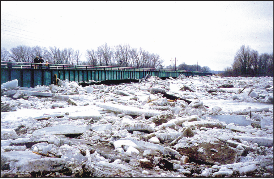
Figure 5. Ice jam lodged against a bridge; Iowa River, a tributary of the Mississippi River
