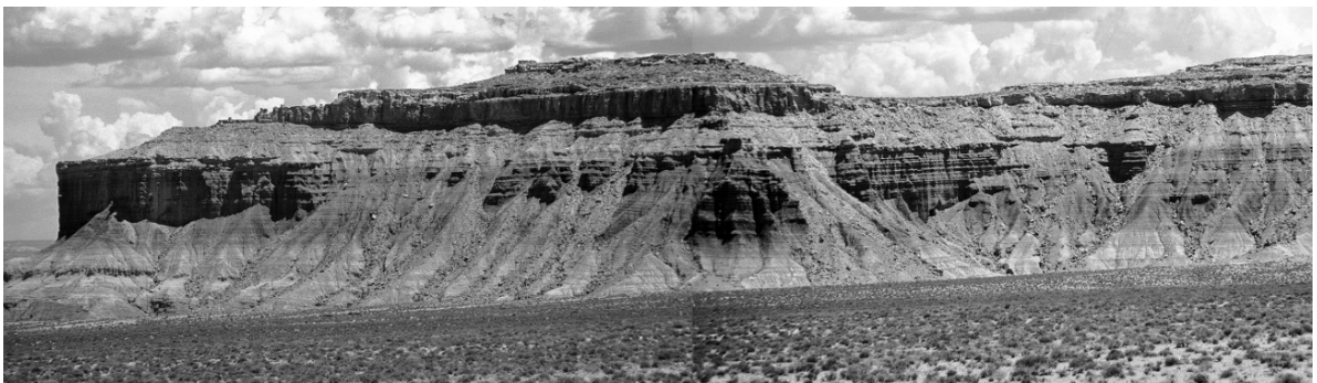
Fig. 8.30 View of northwest face of Goatwater Point, along Utah Highway 95 near Hanksville, Utah, showing rapid backwasting of the sandstones capping the Morrison–Summerville escarpment in the absence of the gypsum caprock. Vertical cliffs
