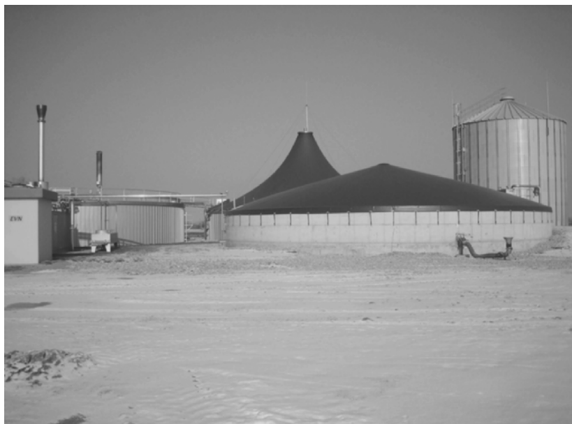
Fig. 13.13. Photograph of a typical two step stirred tank reactor energy crop digestion plant, showing the covered digester storage tank (foreground), a separate gas storage and an integrated gas storage, together with the main digester (Foto by courtesy of Ing. Pfiel, Rohkraft, Reidling, Austria).
