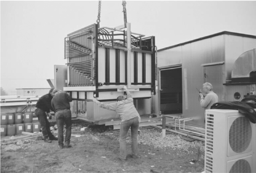
Figure 274. Installation of the dehumidifier
