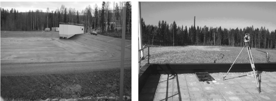
Figure 203. Right: Part of the snow pond with pump house and half of the hospital. Left: Snow covered with wood chips in beginning of the cooling season. Picture taken from the pump house
