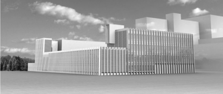
Figure 92. New building of the school of nursing, Sapporo City University (Tentative Name, inaugurated in spring 2006)
