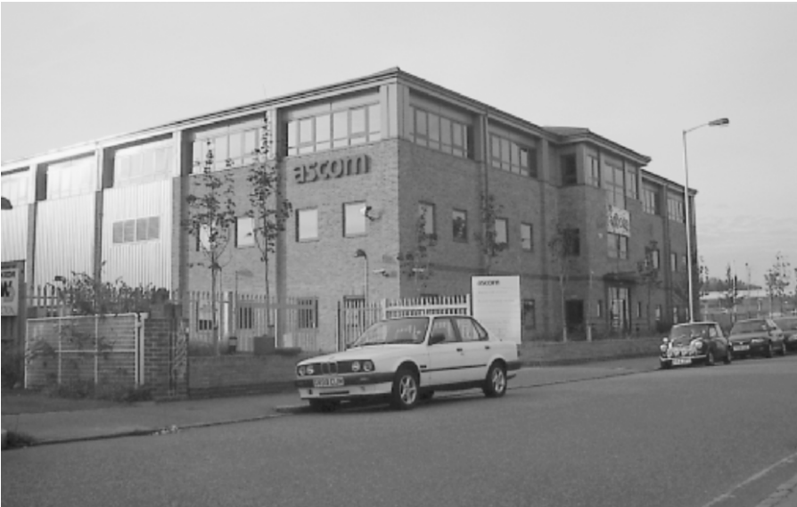
Figure 68. The Croydon building, Commerce way, Croydon Surrey (UK)
