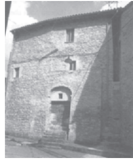
Figure 21. Joint cut between two houses.
