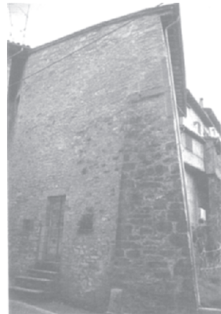
Figure 19. Addition of buttresses
