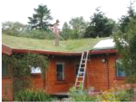
Figure 3. Roof garden house (Eco Village Findhorn).
