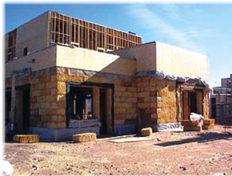
Figure 2. Straw bale construction.
