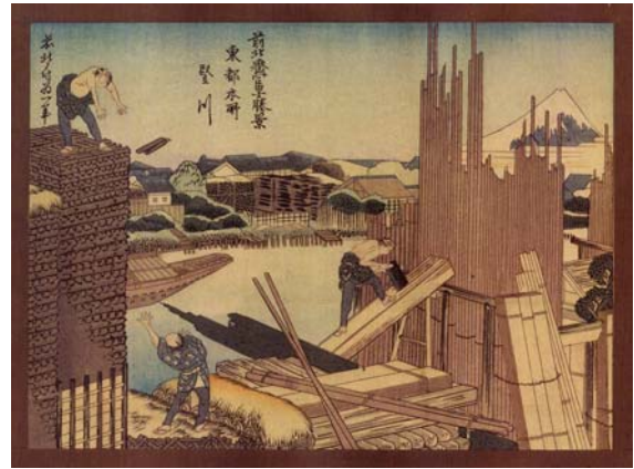
Timber-Handling Technology in Japan. Fig. 1 Stacking wood at a lumberyard on Tatekawa Canal in a harbor side section of Edo (today's Tokyo). Men on the left stack split pieces of fuel wood; bales of charcoal are stored under thatch cover at their feet; sawyer on right rips a timber to form planks; poles are stacked vertically to his right, partially obscuring Mt Fuji; planking, boards, squared timbers, and long green bamboo poles are below him. (Katsushika Hokusai, Thirty Six Views of Mt. Fuji (ca. 1820), in the author's possession.)
