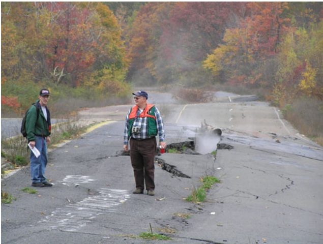
Coal Fire (Underground), Figure 1 Surface manifestation of an underground coal-mine fire includes ground subsidence and smoke, as shown here along a former section of Pennsylvania Route 61 at the Centralia mine fire (Stracher et al., 2006). The asphalt road through the town of Centralia is subsiding into abandoned coal-mine workings, where anthracite is burning underground. A detour was constructed around this section of the highway. Coal fires emit dozens of toxic gases into the atmosphere including carbon monoxide, benzene, and toluene, in addition to green-house gases. Minerals and creosote (coal tar) that nucleate at the surface from coal-fire gas may serve as vectors for the transmission of bio-accumulated pollutants, including Hg and As, from water, soil, and wind-blown dust (Stracher, 2004; Stracher et al., 2005, 2009) (Photo by Janet L. Stracher, 2006).
