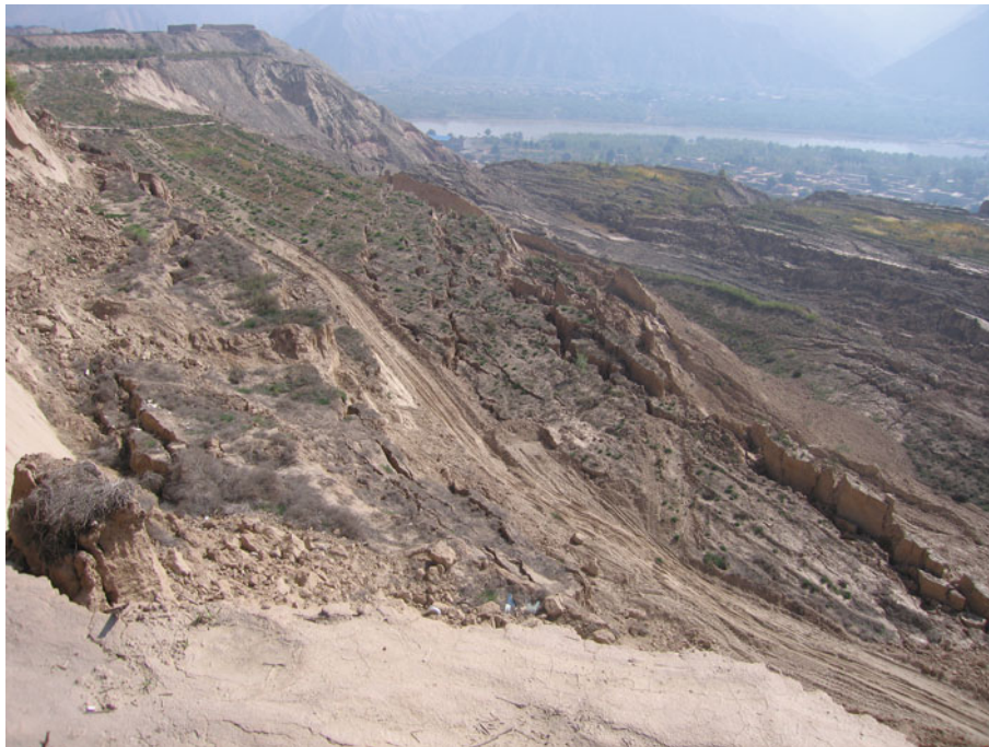
Collapsing Soil Hazards, Figure 3 Complex retrogressive block collapse in thick loess on the fourth terrace of the Yellow River (Huang He) at Heifantai, ca. 60 km southwest of Lanzhou city, Gansu Province, China. Soil collapse has been accelerated by rapid growth of human settlement and resulting widespread irrigation of the terrace for agriculture. The river in the distance is the Huang Shui, here just above its junction with the Huang He. Photograph taken in 2006 (Reproduced with permission from E. Derbyshire).
