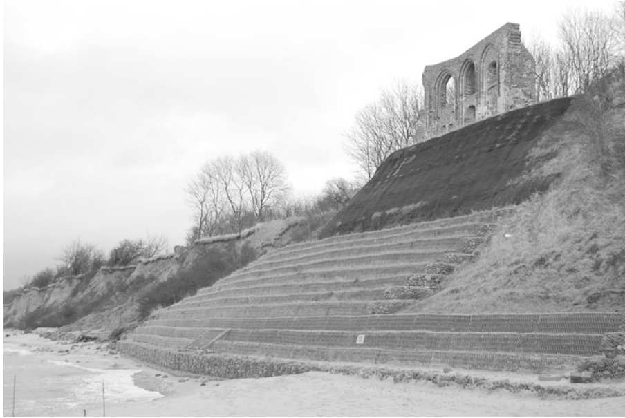
Cultural Heritage and Natural Hazards, Figure 3 The remains of a medieval church in Trzęsacz, northern Poland, atop a Baltic Sea cliff. The church was built in the fifteenth century about 1 km from the cliff edge, but long-term cliff recession resulted in a few successive collapses since 1900. Today the site is considered to be of special cultural importance and protected against further cliff erosion. However, erosion continues unabated next to the site (Photo P. Migoń).
