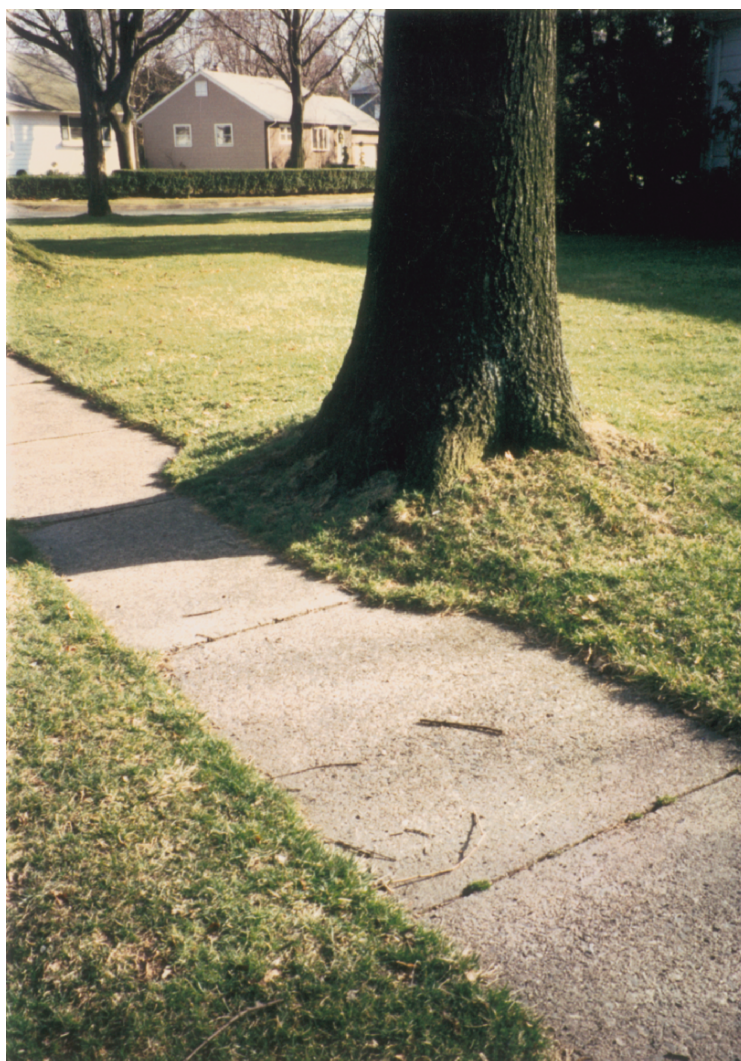
FIGURE 6. Contoured sidewalk creates “breathing room” for the tree. Photo, William R. Comery. Note: For most trees 10 to 12 feet of DeepRoot Barrier will be adequate to protect the sidewalk from future damage.
