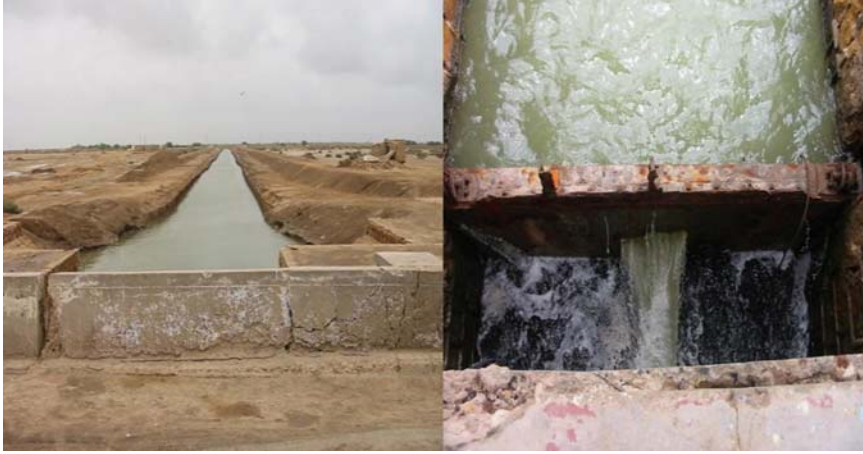
FIG. 5.3.10. Seawater intrusion through the network of canals constructed for the discharge of saline groundwater to the sea.
