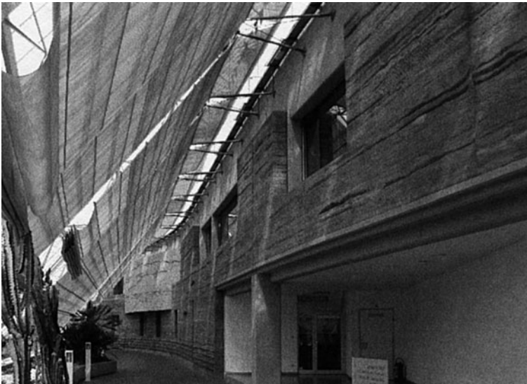
Fig. 8.16 Rammed earth wall, Hospital of Feldkirch, Áustria (Berge 2009)
