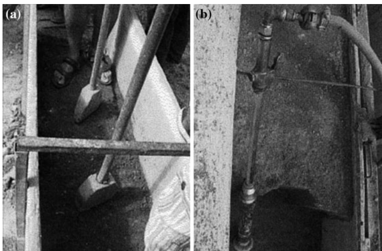
Fig. 8.5 Rammers for earth construction: a Manual, b Pneumatic
