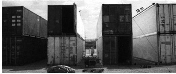
Fig. 10.7 The canyon street pilot site (PICADA 2006)
