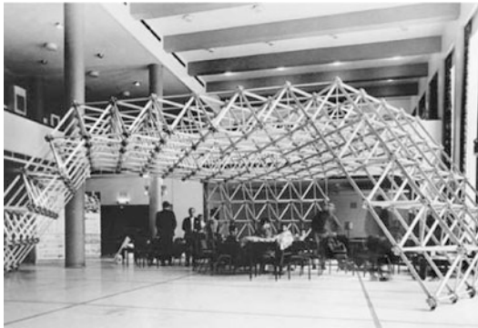
Figure 8.17. "Octet" spaceframe (student project).
