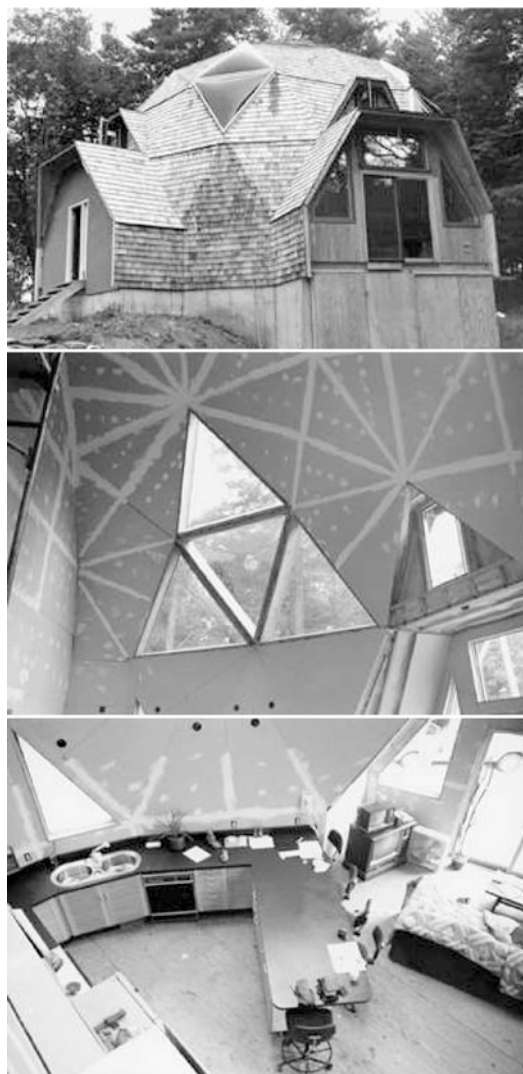
Figure 7.6. Geodesic dome house under construction in Hadley, Massachusetts.
