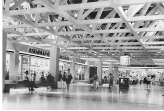
Figure 8.22. Plaza Côtes des Neiges . Shopping center, Montreal. Architects: Mayers and Girvan. Structural engineers: Baracs and Gunther.
