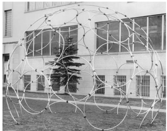
Figure 8.19. Articulated ring-dome (student project).
