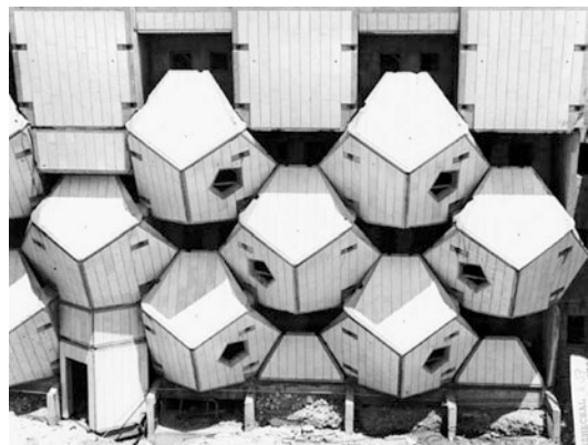
Figure 7.11. Housing complex in Ramot, Israel, 1972–1980.
