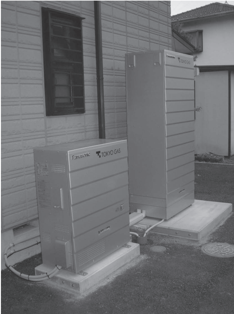
Fig. 1 Residential polymer electrolyte fuel cell cogeneration system operated in a customer's house
