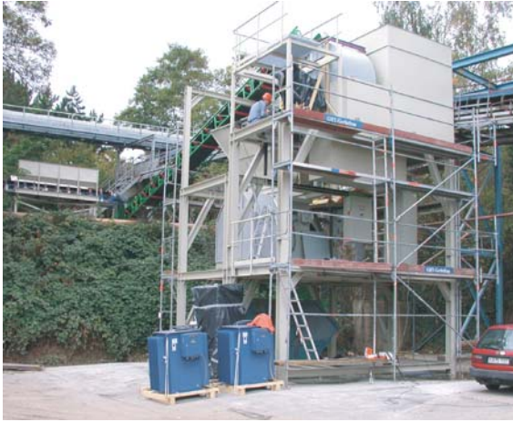
Fig. 17 Prototype facility KEA-ZAR during construction at the factory site
